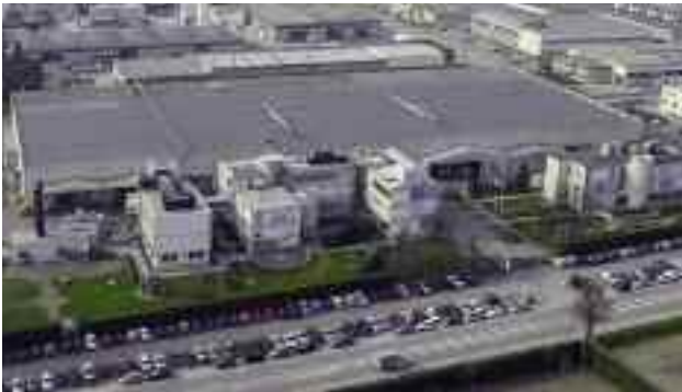
Emerson Network Power Headquarters EMEA
